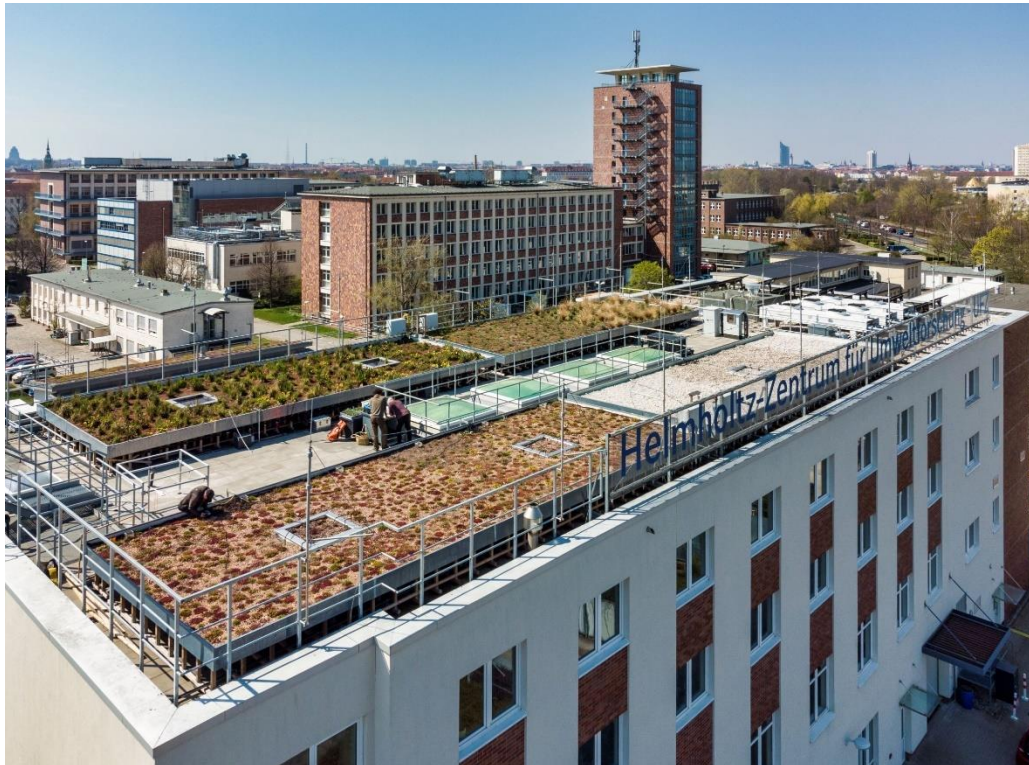
Figure 2 – Show the green roof test center in Leipzig
