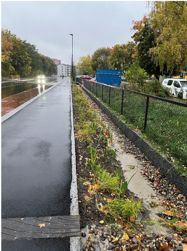
Figure 6 – Show a part of the raingarden project in Oslo
