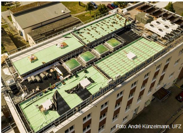
Figure 3. Green roof for rainwater retention and storage for reuse in Leipzig, Germany. Image: André Künzelmann (UFZ). Source: multisource.eu
