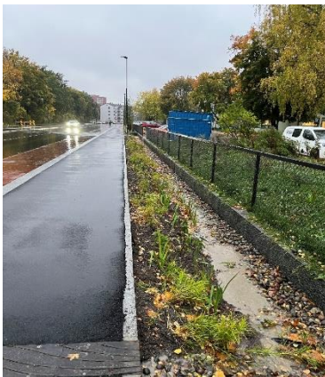
Figure 2. Raingarden for road runoff treatment in Oslo, Norway. Source: K Karlstrøm, 2022.
