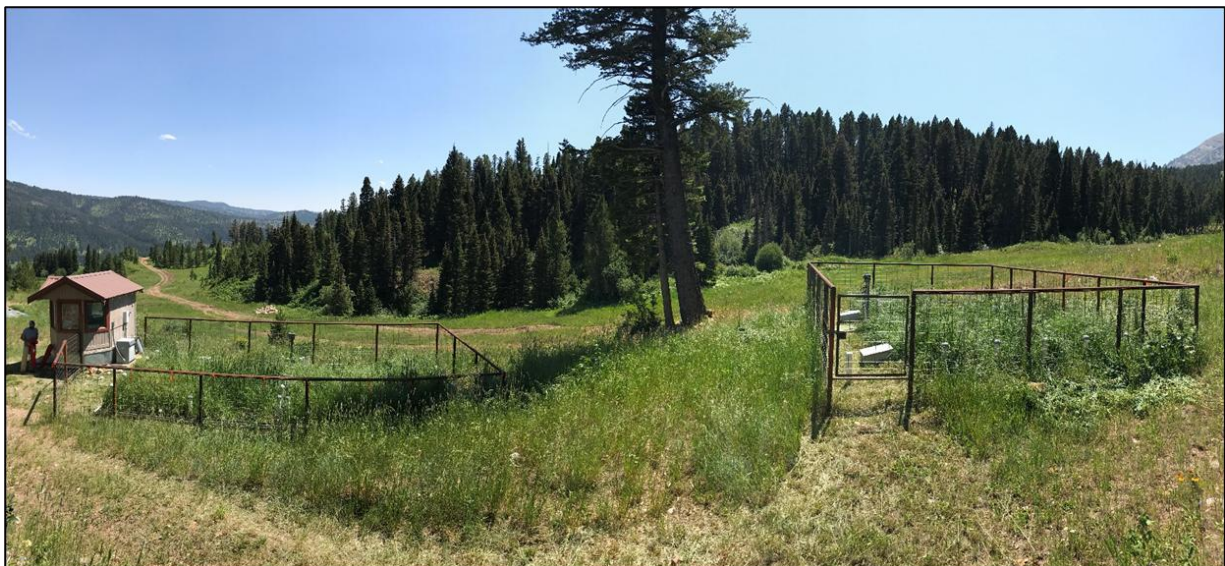
Figure 3.3. Photographs of the Bridger Bowl TW pilot system. Top – photo in summer, showing both stages of the system within the fenced areas and growth of Carex and Phragmites . Bottom left – System in winter, with two pilot system stages enclosed within two rectangular fenced areas on left side of the photo. The full scale treatment wetland is within the larger fenced area behind and to the right. Bottom right – closer view of the second stage of the system in winter.
