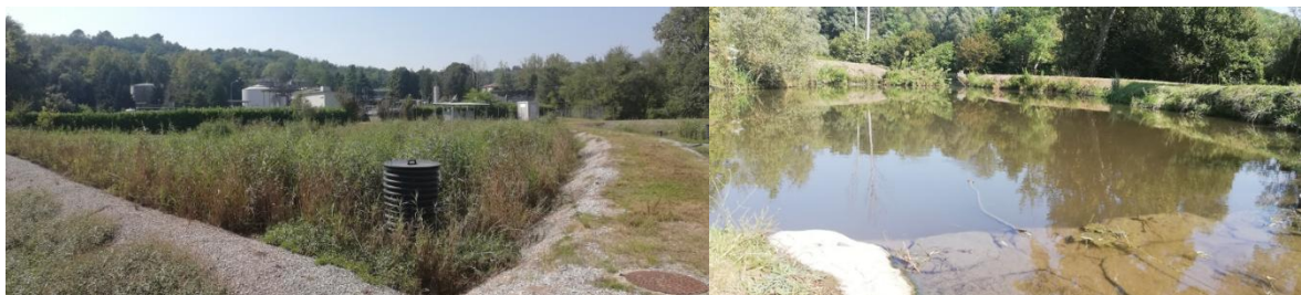
Figure 5.3 Picture of the Merone hybrid treatment wetland, aerated wetland (left) and polishing pond (right). Site visit: September 2023.
