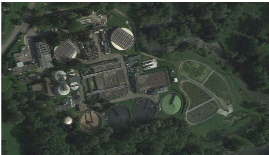
Figure 5.1 Demo 4 of Merone aerial view. Source: Google Earth.
