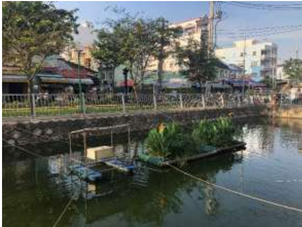
Figure 8 Site visit: Floating Treatment System - HCMC canals
